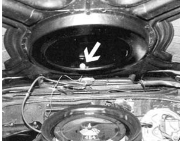
Air flow valve solenoid is visible (arrow) inside hood. This is the opening that the air cleaner seals shut.
